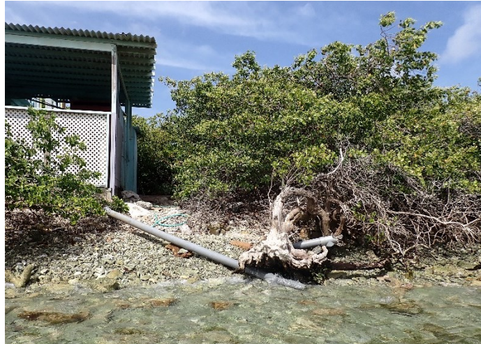
Image 11: Sewage pipe from Rancho dumping directly into the sea.
