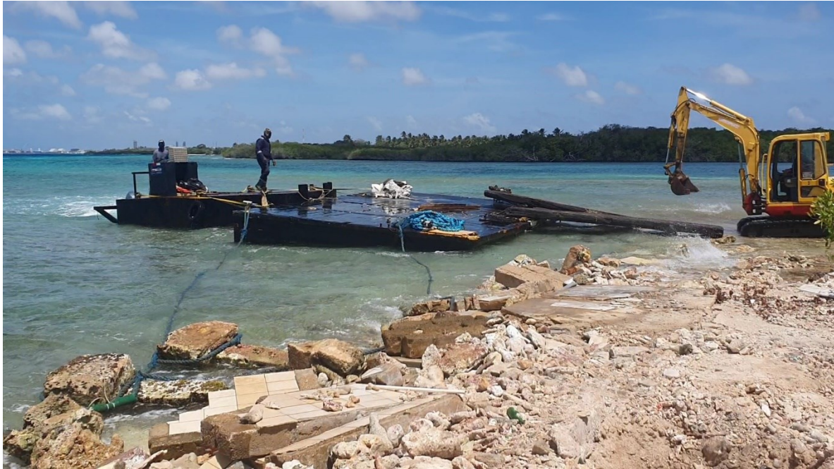
Image 16: Excavator in position to move onto barge
