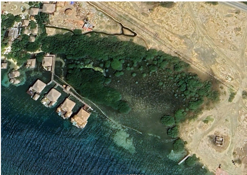
Figure 7. The area under management by FPNA and the adjacent Aruba Ocean Villas development, Google Earth image of April 2023 (12.26'37"N 69.56'31"W).
